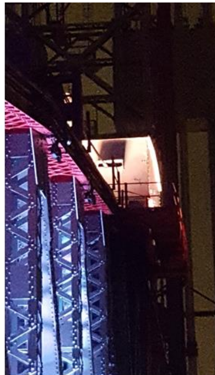
Lighting to main span with Wheelhouse illuminated in the background
