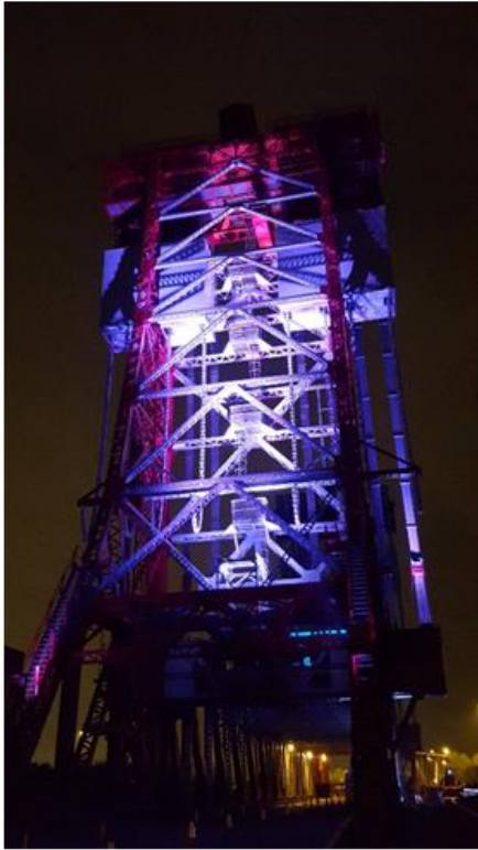
Lighting to main tower mainly internal illumination with additional lighting to outer elevations
